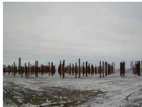
The hospital's pile foundation was constructed by UICC.
