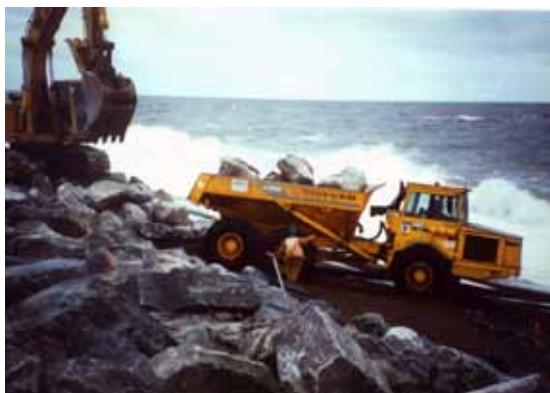
Pt. Hope Seawall
