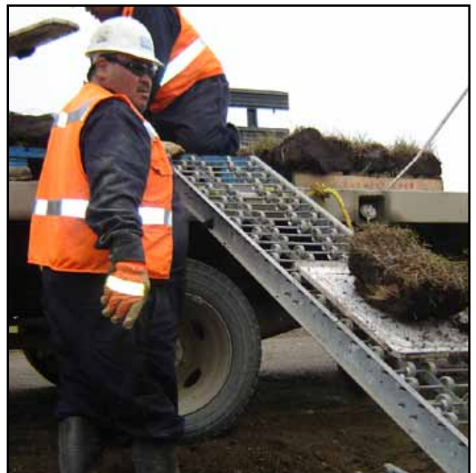
UIC shareholder Jens Hopson Jr. moves pieces of sod using a roller conveyor system.
